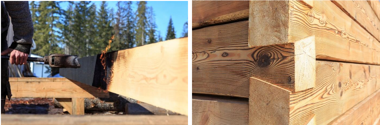
Torched timber seals the pores of the wood and highlights the grain lines in the timber.
